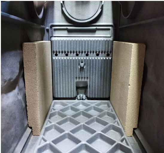
1. Slide the side plates until the back of the stove
